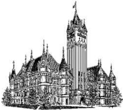
SPOKANE COUNTY COURTHOUSE
